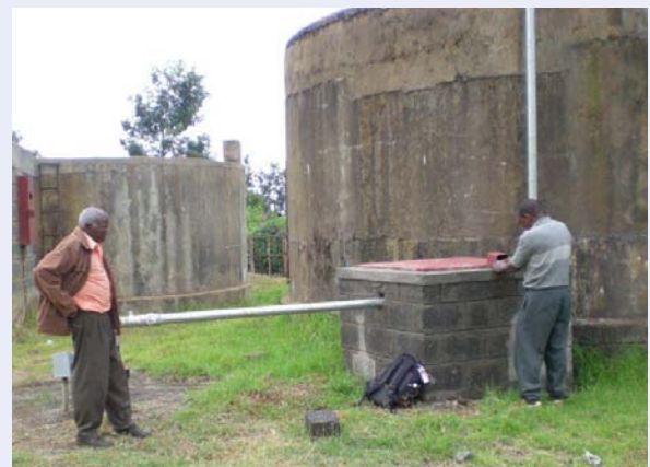
Storage and distribution tanks at Karaweti Water Project in Githunguri division of Kiambu district. The community borrowed $50,000 from K-Rep Bank to develop a new source and install meters for all its customers. As a result, revenue collection increased by 90% and the reliability of water services increased tremendously, with 87 percent of customers receiving water seven days a week, up from 8 percent before the investment.
