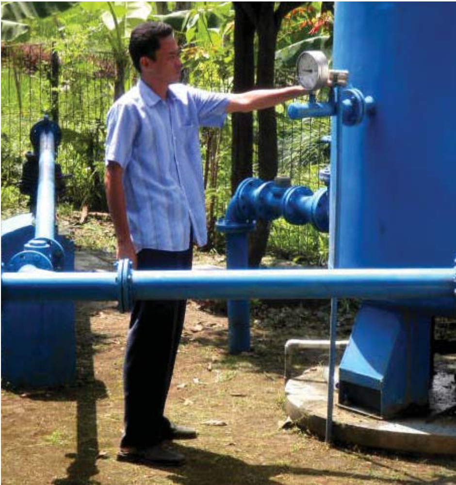
Illustration 4 : Checking Out Water Pressure in Cianjur, West Java
