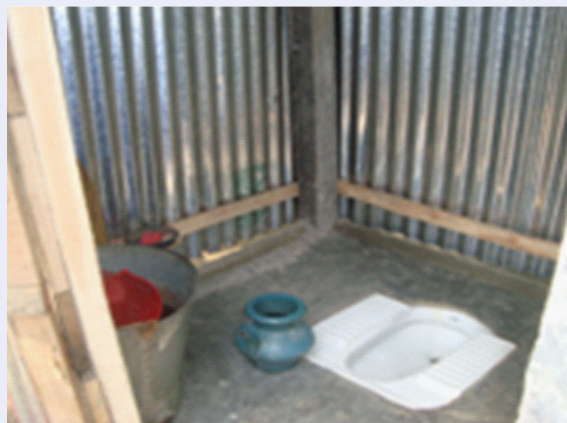
Improved toilet. Cost: US $60.
