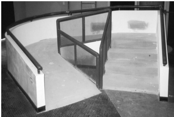
Stairs and Ramp: City Room
