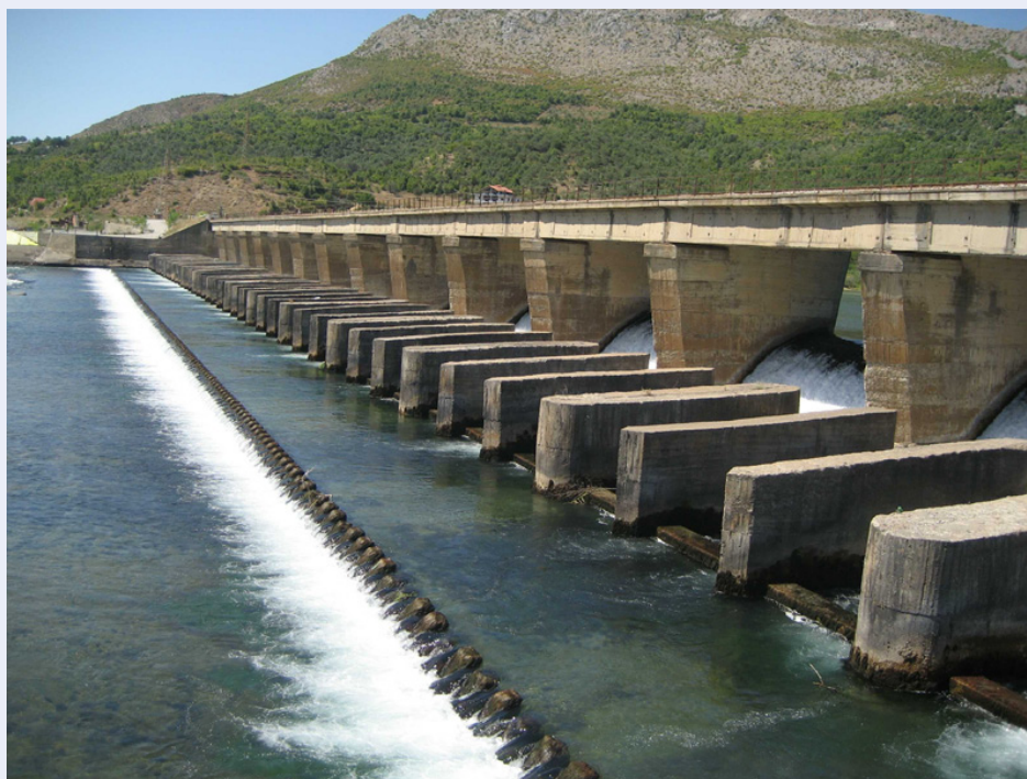
The Ashta run-of-river hydropower plant weir. (Photo by Tullio Marrama)
