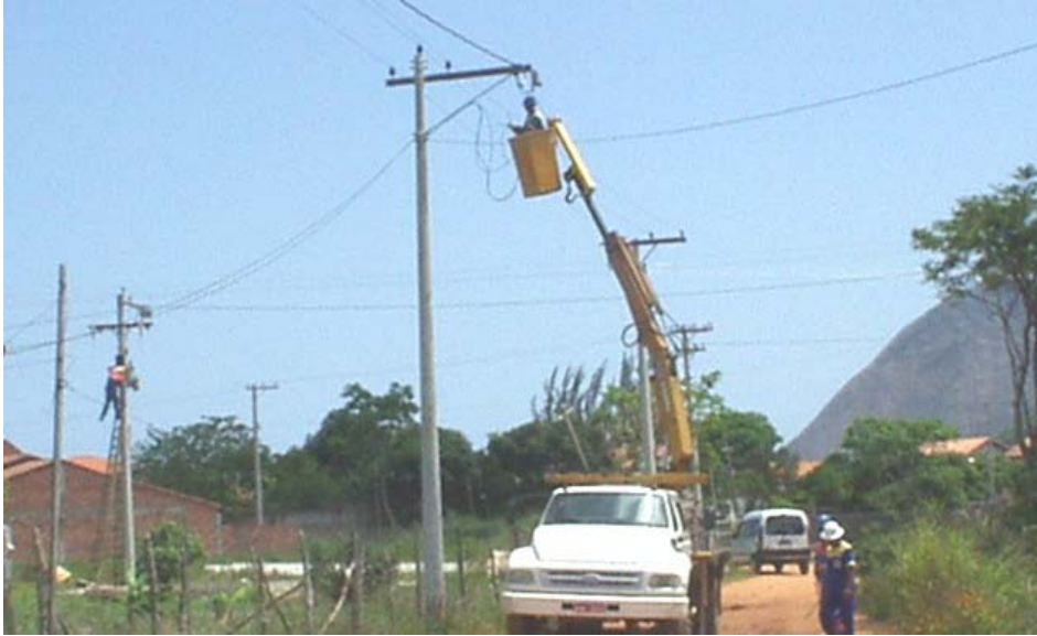
Figure 5: Typical MVD arrangement
