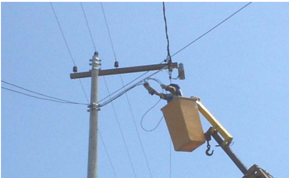
Figure 6: Shielded connections in MVD
