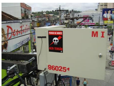
Figure 6.5: SENTINELA - AMI solution to reduce non-technical losses in supply to low voltage large consumers
