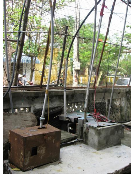
Informal connection of water pipes
